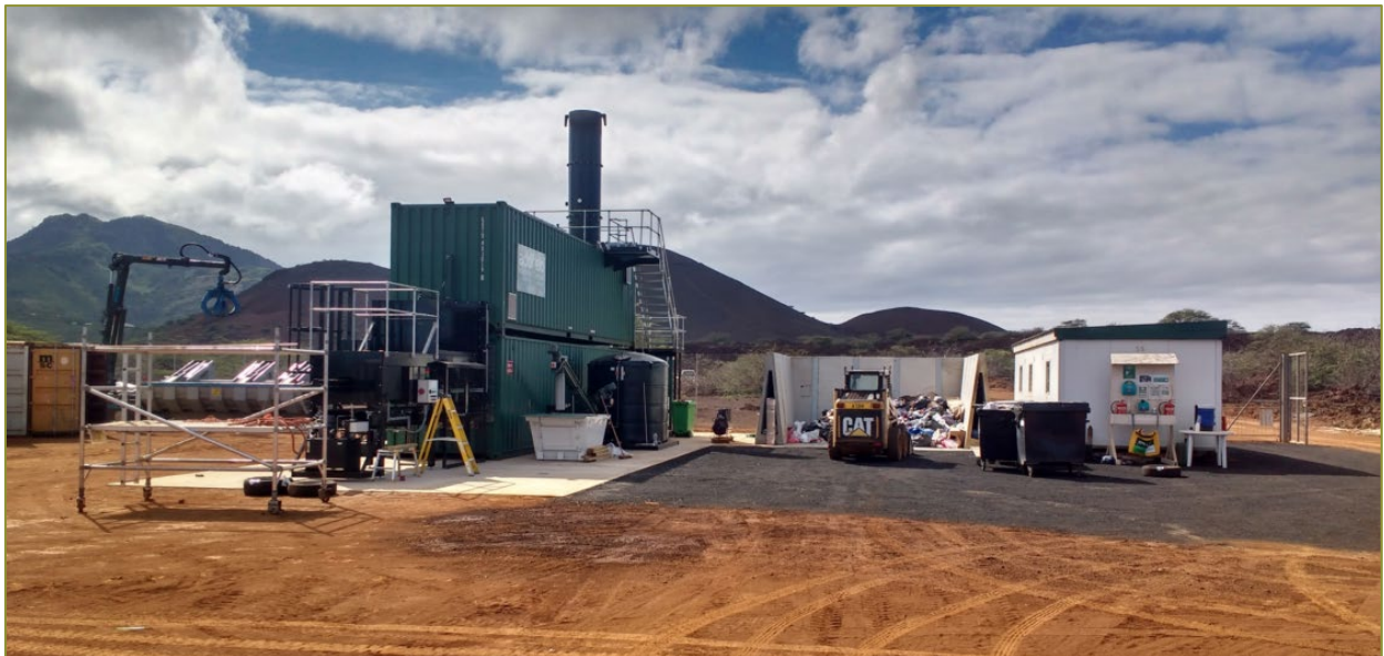
Figure 5 - One Boat HWRC in Construction Photo
